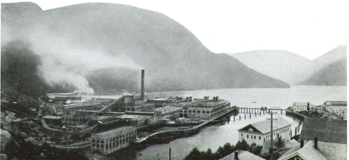
The huge pulp and paper plant at Ocean Falls, B.C.
