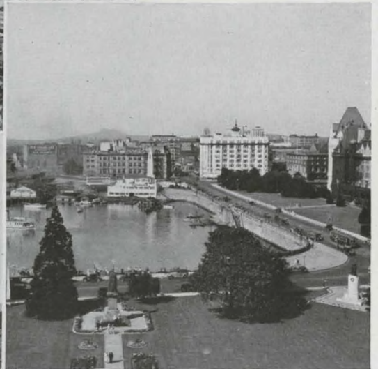
Top: Vancouver, from the air. Centre—left and right: Parlia- ment Buildings and view of Inner Harbour and Govern- ment Street, Victoria.
