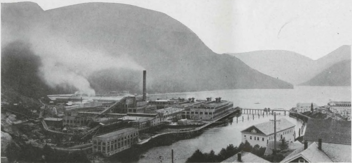
The huge pulp and paper plant at Ocean Falls, B.C.
