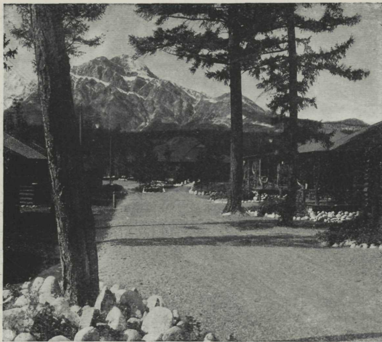
The rustic bungalows are steam heated.
