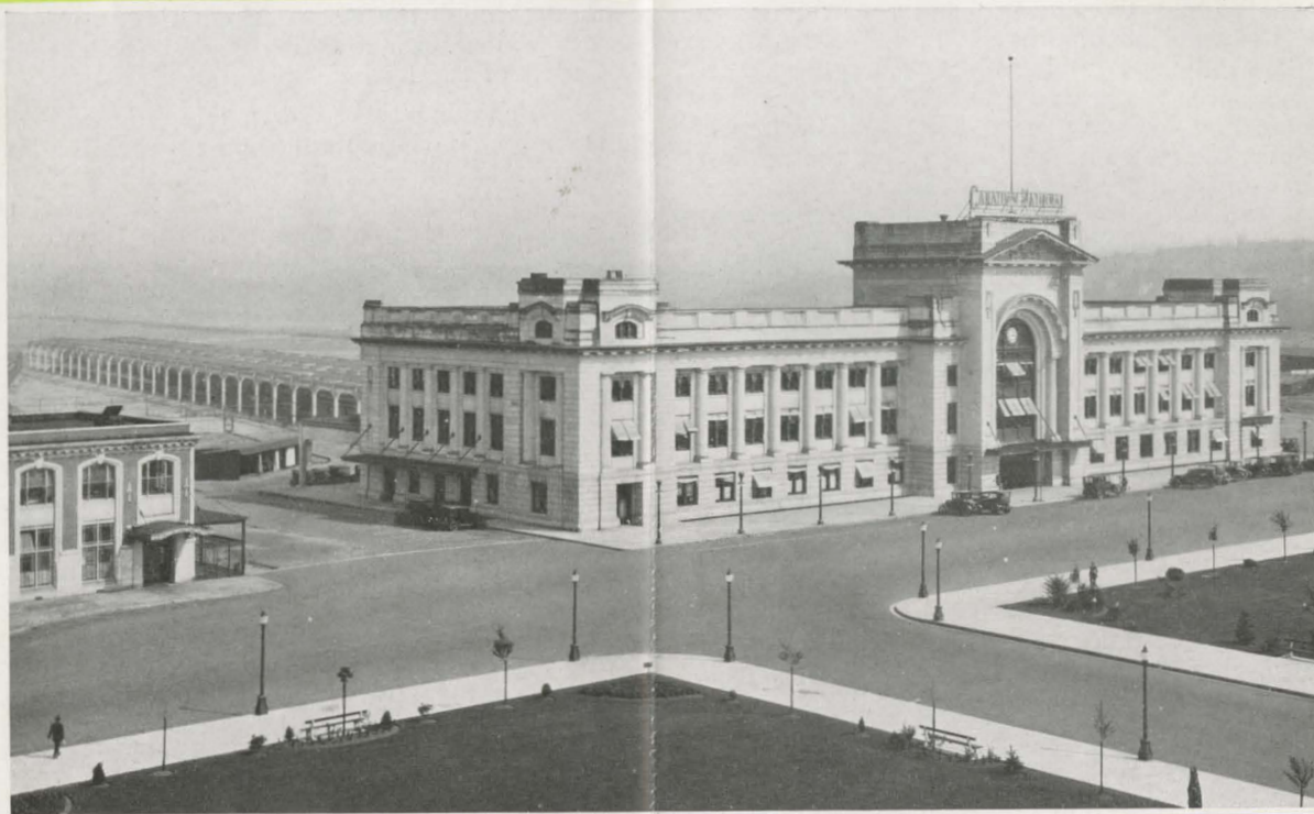
Canadian National Railways Terminal—Vancouver.
