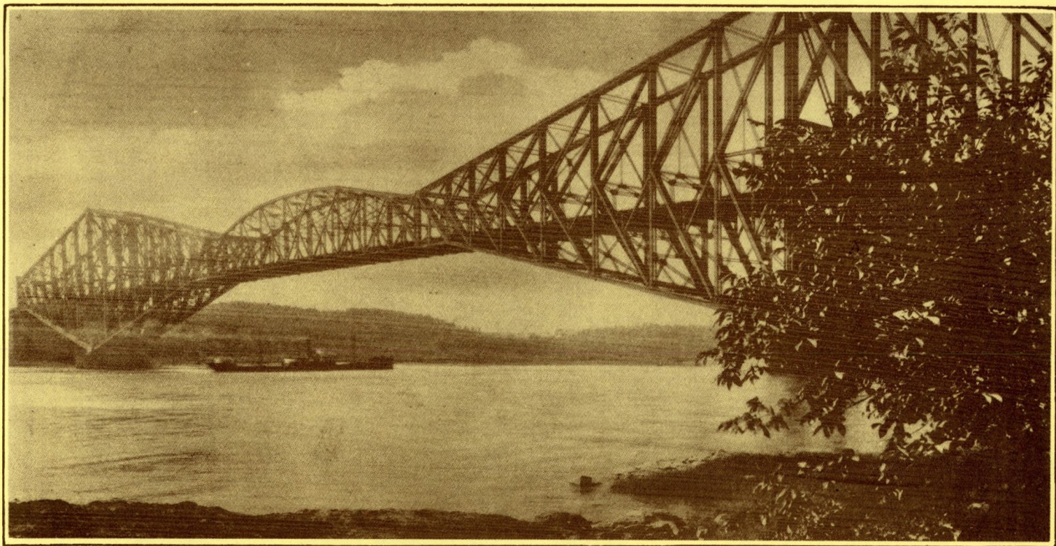
The Quebec Bridge of the Canadian National System. Its main span, 1800 feet, is the longest in the world, being 90 feet greater than that of the famous Forth Bridge in Scotland
